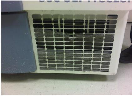
Dust or grime buildup on the filter (Figure 6) blocks the normal air flow through the condenser, which reduces the ability of the ULT freezer to effectively dissipate heat. Any air flow that bypasses the clogged filter will result in air carrying dirt to deposit on the condenser. Dirt on the condenser increases energy used in the compressor to transfer heat to the ambient environment.
